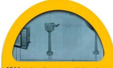
**1966:** At Dum Dum airport (Calcutta) was installed Transmissometer to assess the runway visual range (RVR).
